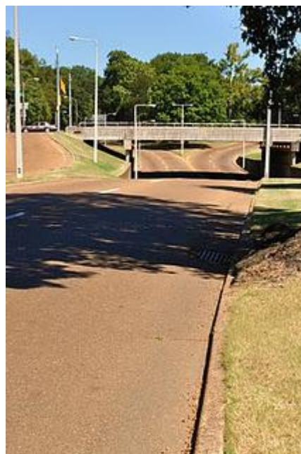
Union Ave, underpass on East Parkway
